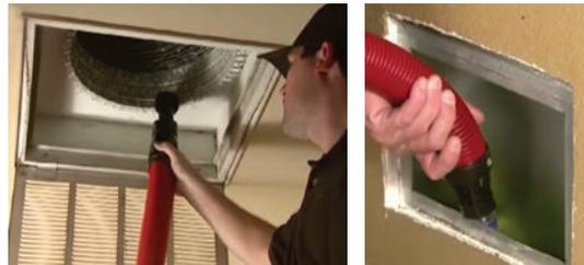
Our Rotobrush spinning brush and HEPA\* filtration system ensures a clean environment during and after cleaning.
